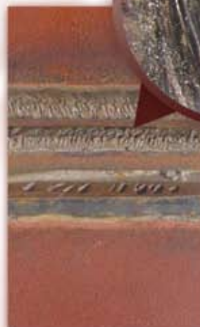
Fracture of weld seam without suitable welding primer
